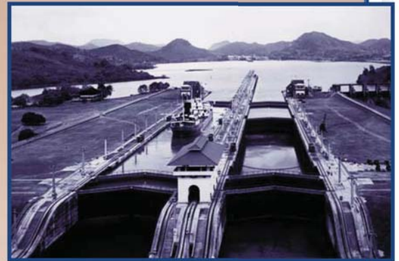
▲ This photo shows a ship that has entered the canal from the Pacific Ocean side and is heading north through the Miraflores Locks. Ships and boats can also enter the canal through the Atlantic Ocean side and head south through the Gatún Locks.
